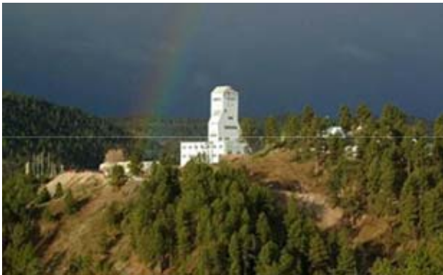
Figure 6, Homestake Mine Shaft Head House
