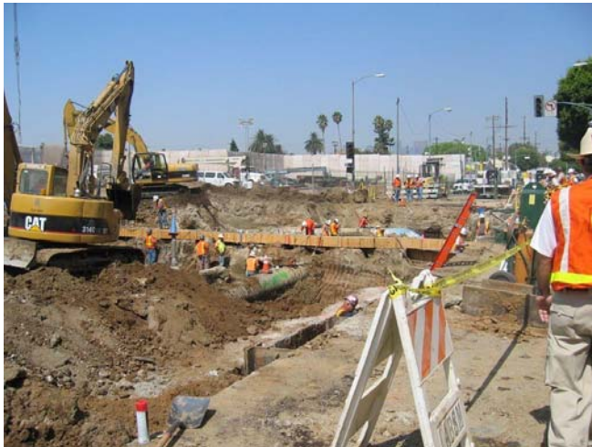
Figure 2, Cut and cover construction, Los Angeles, CA
